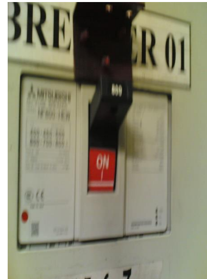
Replaced : Circuit Breaker 62kAIC Circuit Breaker
