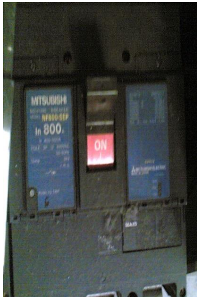
Installed 42kAIC Circuit Breaker
