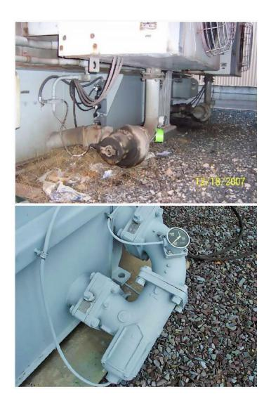
If the case of transformer that has Oil pump(s), maintenance staff must check flow indicators and pump isolation valves to ensure oil is circulating properly.
