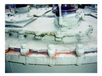
Oil leak is very dangerous, especially if not spotted on time. What should maintenance people would do? They should check the entire transformer for oil leaks. Leaks usually develop due to gasket wearing out. Ultraviolet exposure, or from expansion or contraction, especially after transformer have cooled, due to thermal shrinkage of gaskets and flanges.
