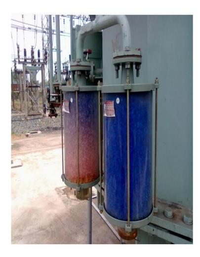
Check the dehydrating (desiccant) breather for proper oil level if it is An oil type unit. **Check the color of the desiccant** and replace it when approximately one-third remains of the proper color.
