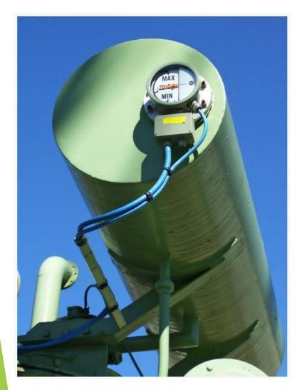
This gauge indicates oil level by displaying A temperature. Compare the indicated temperature on the conservator level gauge with The top oil temperature indicator. They should be Approximately the same.
