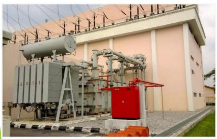
If the transformer has a nitrogen blanket, **check the pressure gauge for proper pressure**. Look for the operators recording of pressures from the Pressure gauge. If does not change, the gauge is probably defective.
