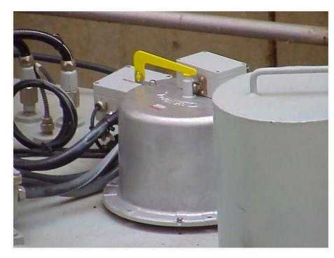
Figure shows a pressure relief device With the yellow indicating arm. With the Transformer under clearance, check the Pressure relief device indicating arm on Top of the transformer to see if has operated.
