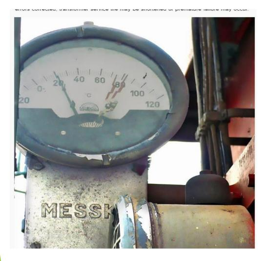
The winding temperature indicator should be reading approximately 15 degrees above the top oil temperature. If this is not the case, one or both temperature indicators are malfunctioning. High temperature may mean overloading, cooling problems, winding problems, core, or connection problems.
