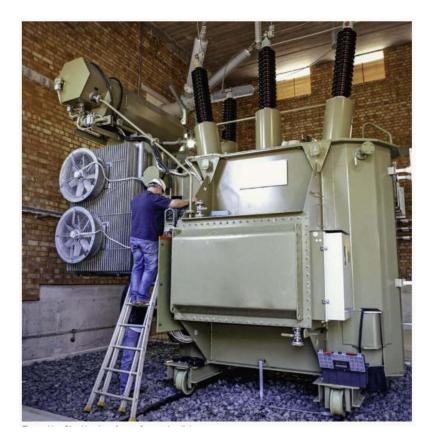
Maintenance staff must check and test all isolation valves at the top and bottoms of radiators to ensure they are open. Inspect cooling fans and radiators for cleaning and fans for proper rotation. Checking for dirty or damaged fan blades or partially blocked radiator is obligatory.
