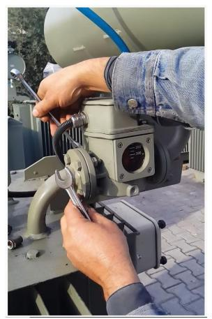
Inspect the isolation valve on the Buchholz relay to ensure it is open. When the transformer is offline and under clearance examine the Buchholz relay by lifting the window cover.
